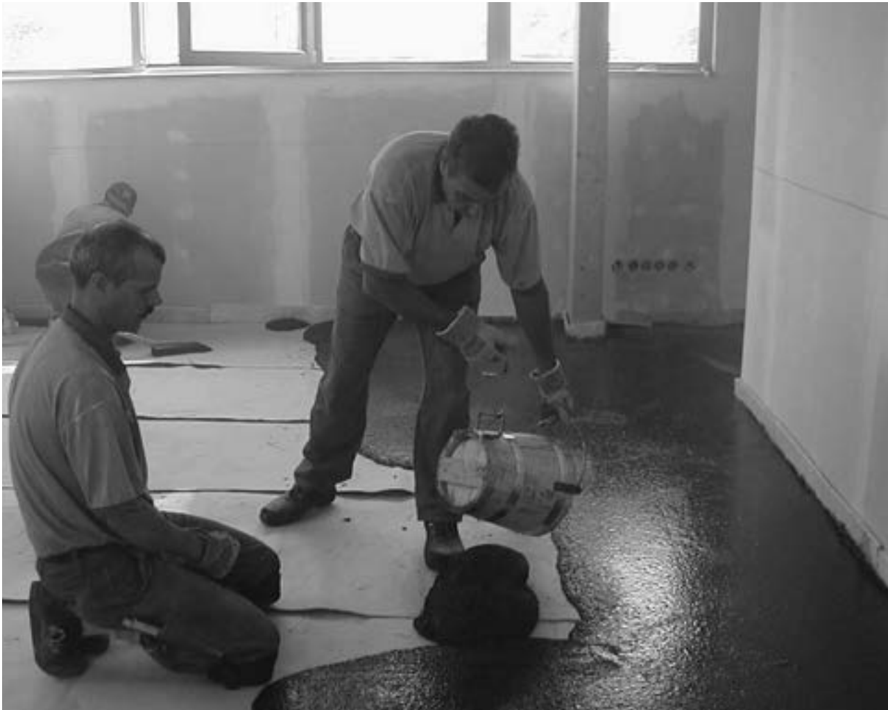
Fig. 1.5 Example of mastic-asphalt application
