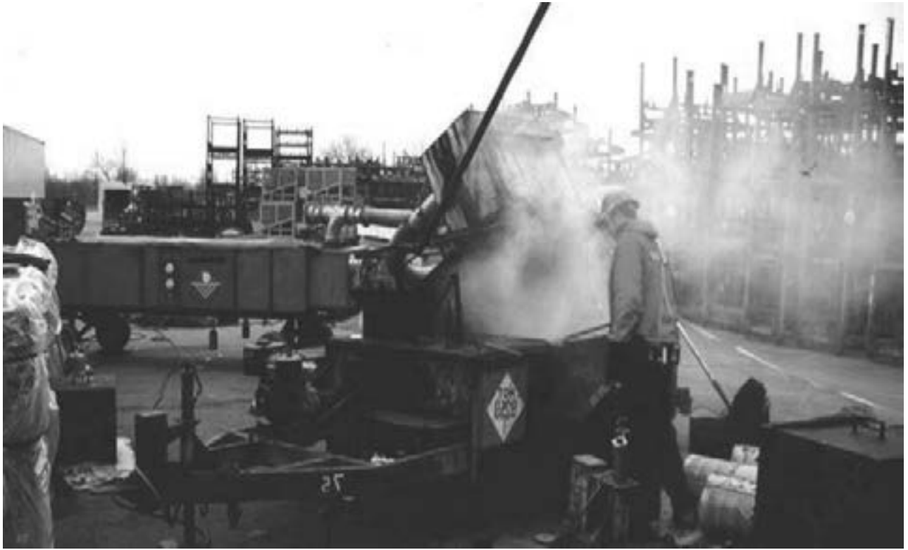
Fig. 1.4c Example of hot-applied bitumen (kettleman)
